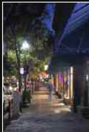
A recent lighting upgrade on Durango's historic Main Street is expected to result in a $3,000 reduction in the city's annual electric bill.
